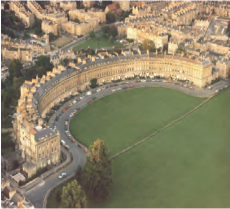
Figure 5.66: Bath Crescent , England , example of crescent shaped building.
