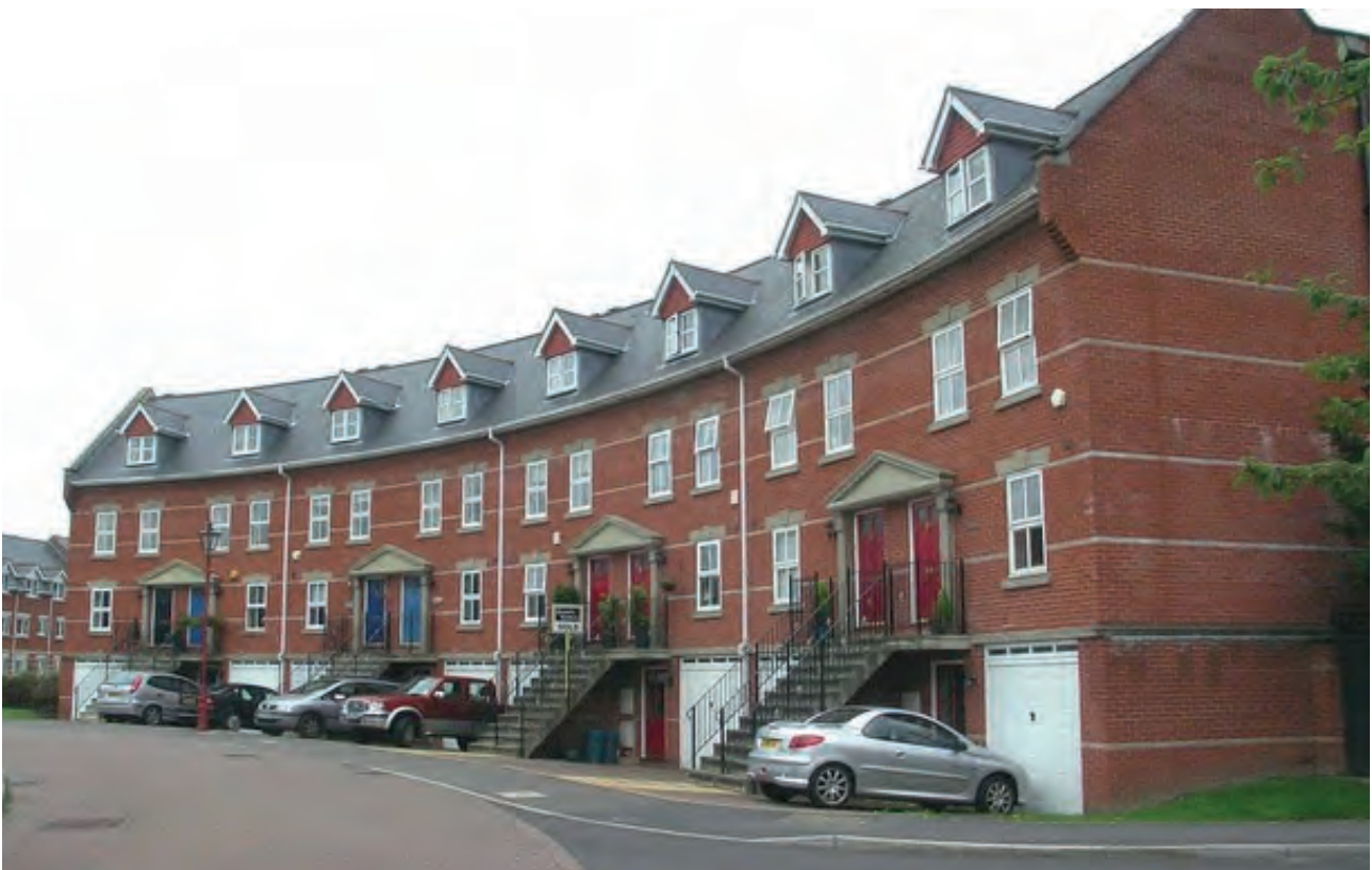
Figure 4.86: Fairmile Crescent, England
