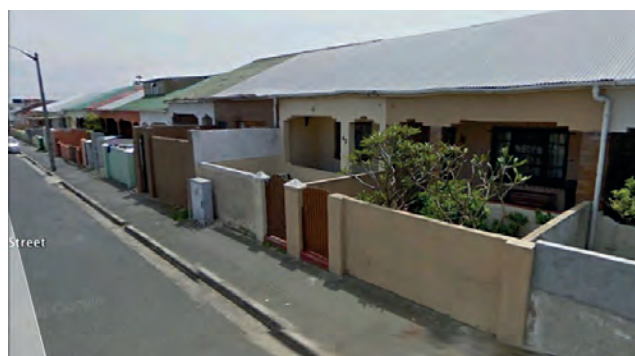
Figure 5.90: Justin Street Row Houses
